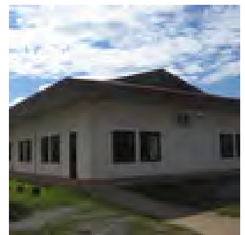
Dining Facility Building
